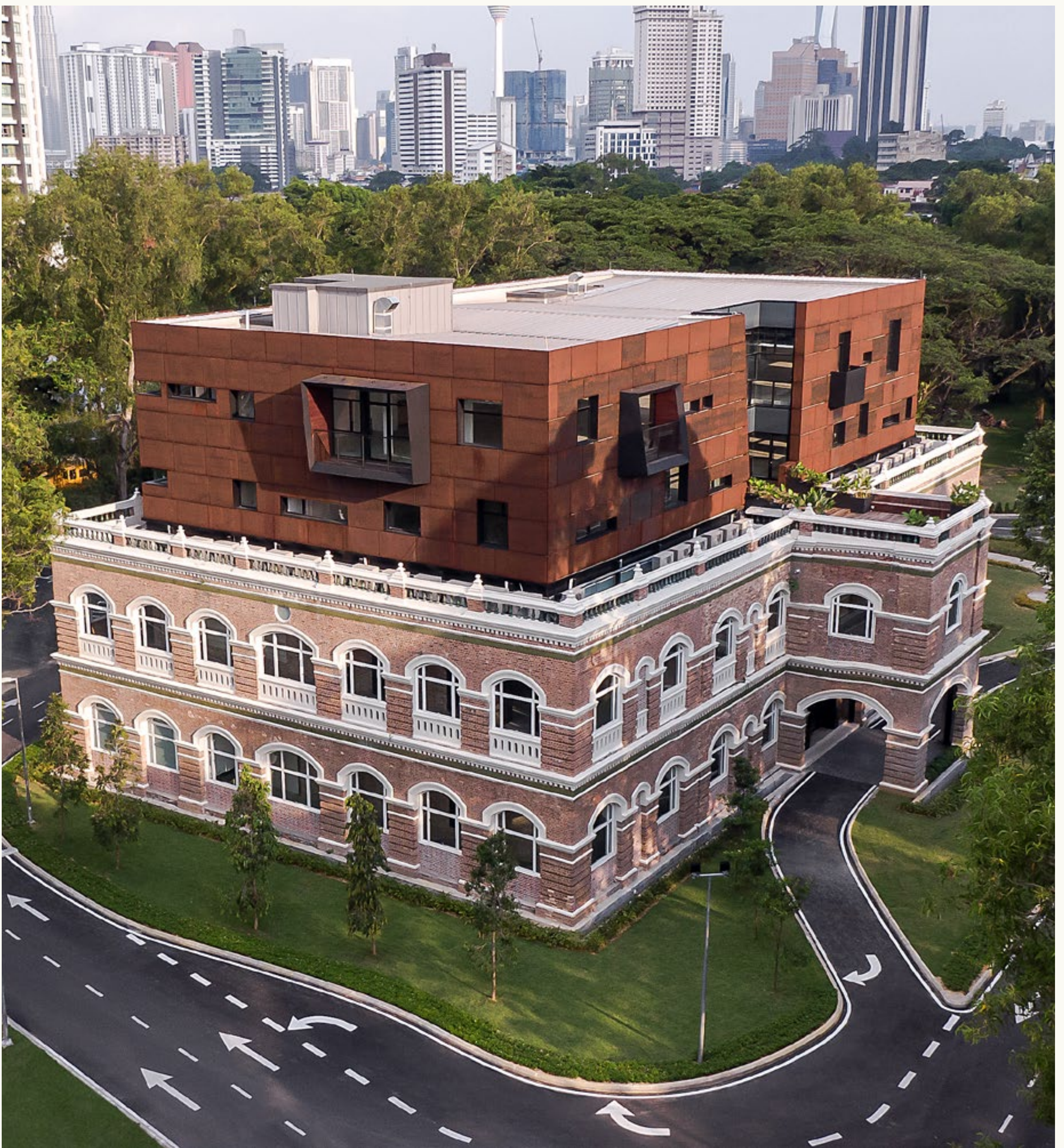
Sentul Works at Sentul West. The historical landscape at Sentul inspires the new, as an old colonial structure provides a canvas to create timeless appeal.
